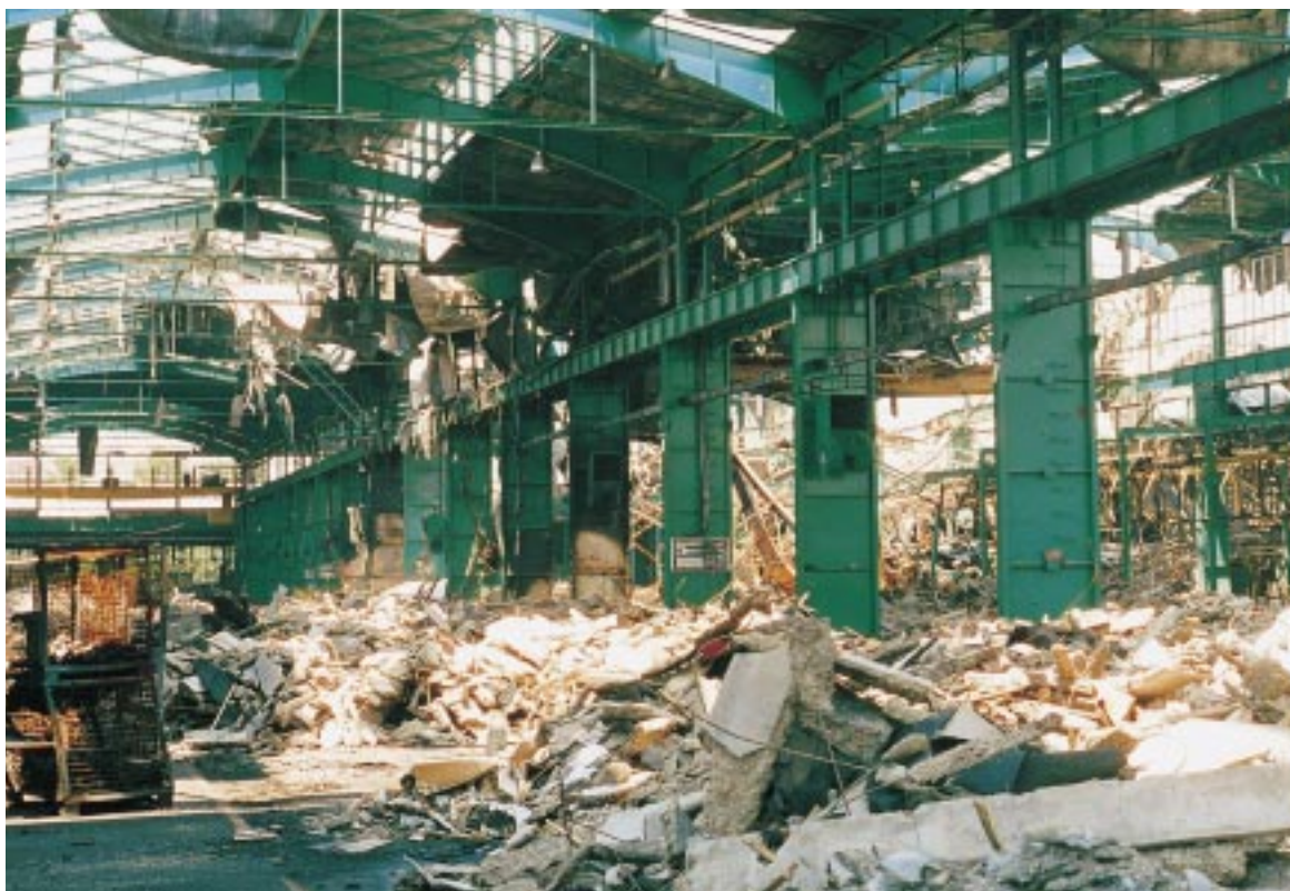
Destroyed factory hall, Kragujevac
