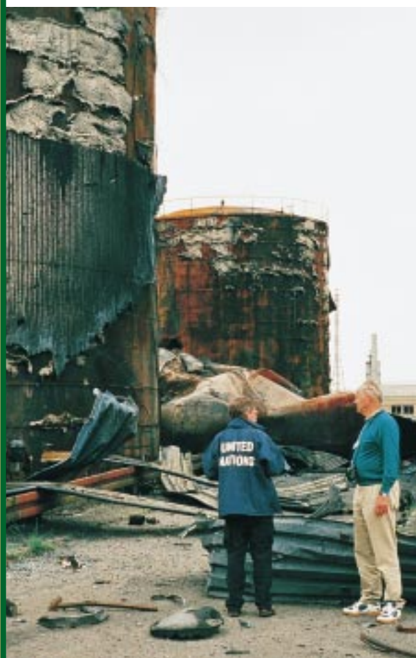
Inspection of damaged oil tanks
