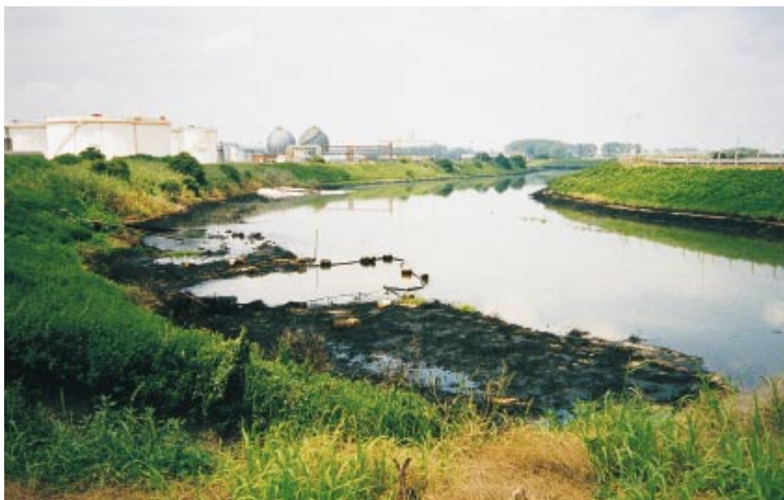
The wastewater canal at Pančevo which flows into the Danube River
