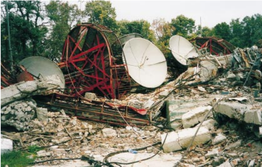
Telecommunications facilities located in Fruška Gora National Park were destroyed during the air strikes
