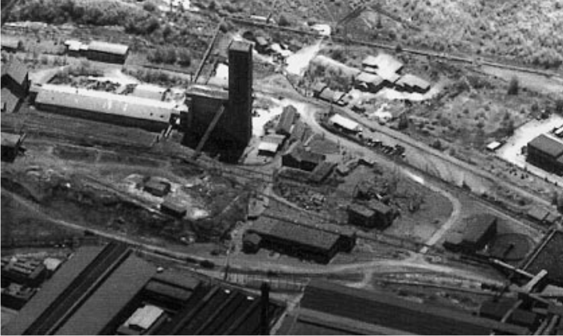
Bor copper smelter and refinery
