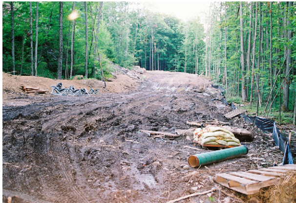
Drilling requires the clearing of land which alters the landscape. Here, trees have been cleared to build a road to reach the drilling site.
