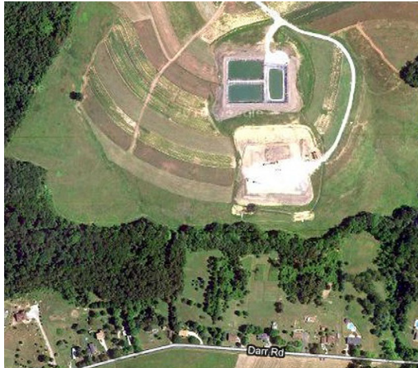
Pools of fracking fluid located few miles away from residential area.
