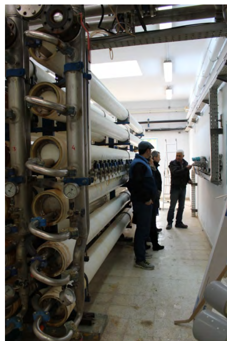
Figure 5 Water treatment plant using reverse osmosis (photo UNEP/GRID-Geneva, 2015)
